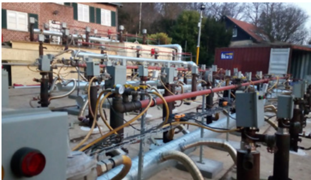
Figure 1. In-Situ Thermal Desorption of hydrocarbon-impacted soil in residential area.
